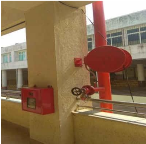
Snap. 2 Water pipeline in case of emergency fire break out near Workshop
