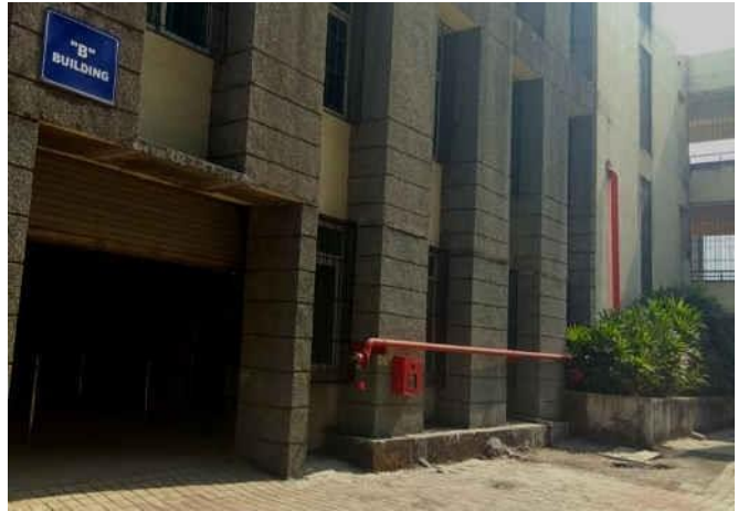
Snap. 2 Water pipeline in case of emergency fire break out near Workshop
